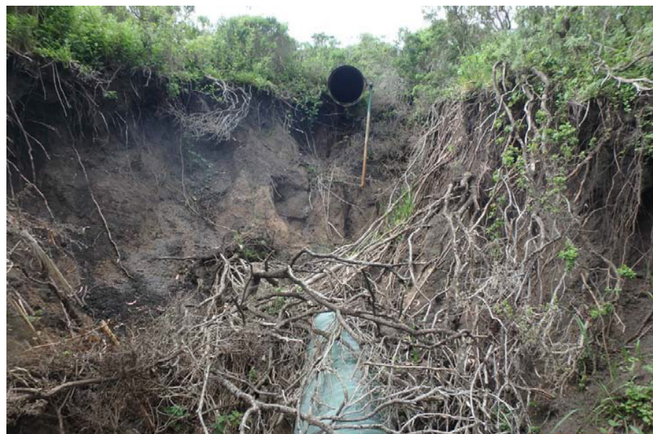
Erosion repair example
