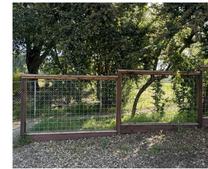
hogwire panel fence 5' or 6' tall, 2x4 frame with 2x6 top, 4x4 pressure treated post and 1x1 picture frame around wire panel
