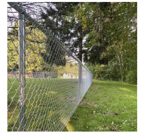
chain link fence
