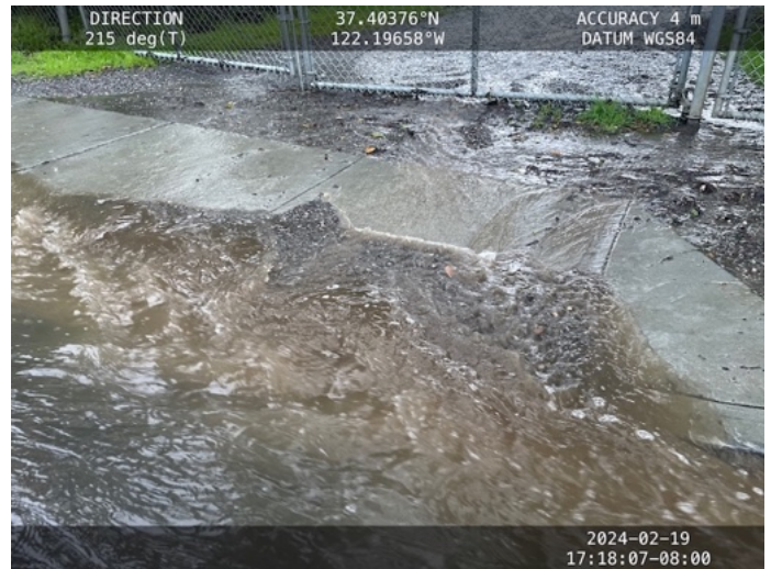
Water flowing onto La Cuesta from the fire access road showing accumulation of gravel driven by flows on access road.
