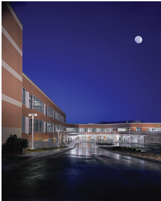
San Mateo Medical Center's Hospital
