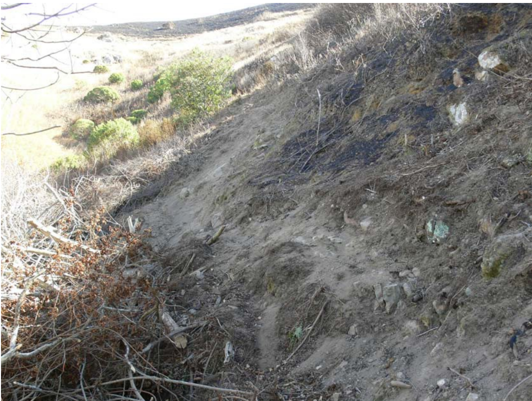
Figure 6. Northeast side of burn area, within a steep ravine. Area was hand cut, and the fire break has created exposed, loose soils. Photo date: 09/20/06.
