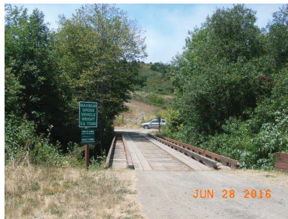
Figure 3. View westward of riparian woodland along both sides of existing bridge.
