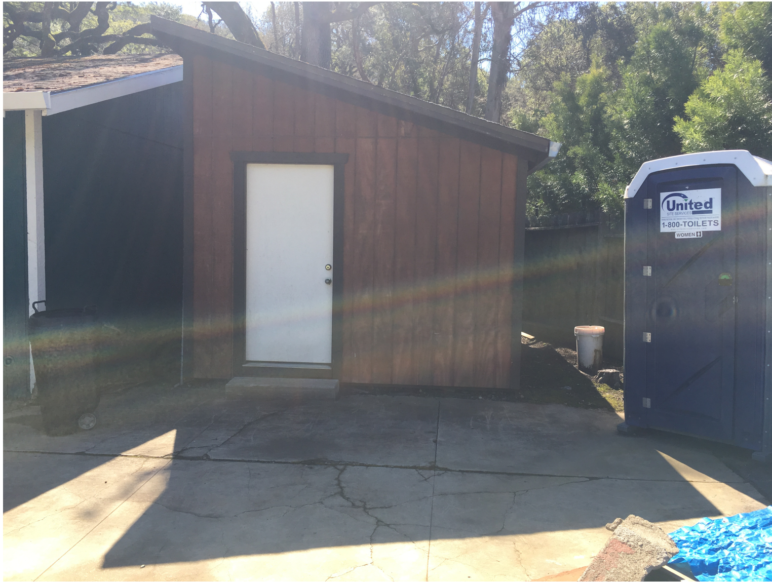
Shed to be removed
