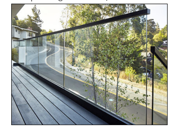
Deck Railing Tempered glass with Ipe handrail
