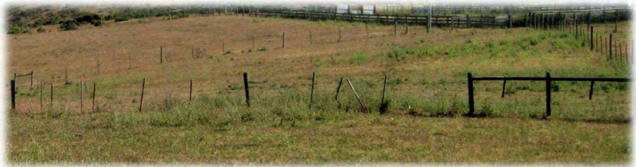
**Figure-9:** Sample of New Zealand style smooth wire fencing on the Toto Ranch. The high tinsel smooth wire is susceptible to damage and often breaks. Most fences on the ranch are older and in varying condition.
