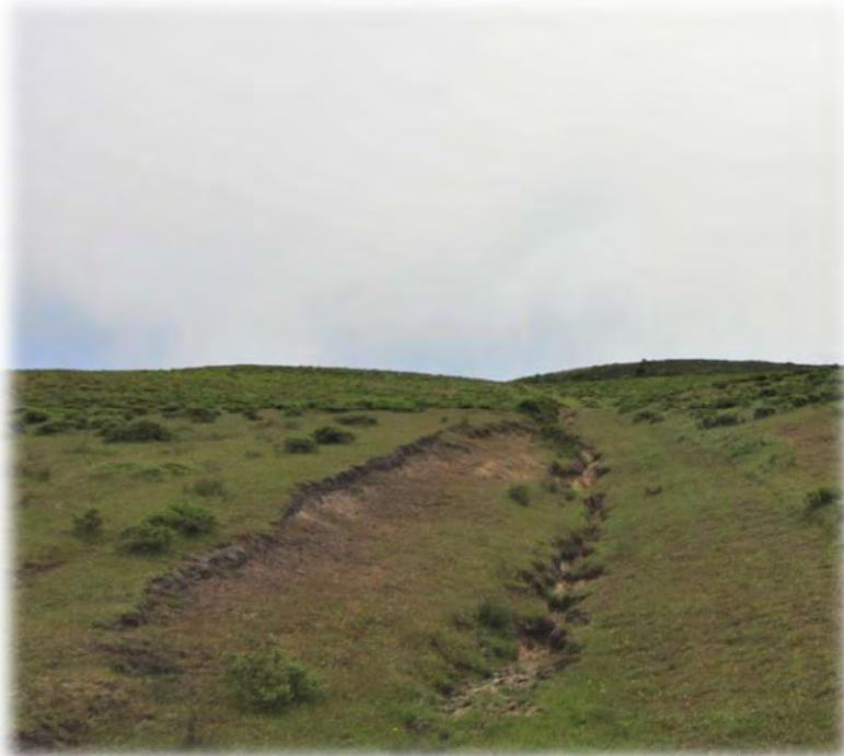
**Figure-8:** Gully/rutting activity along an insloped road just south of the Agricultural Lease area. Large gully caused by surface water flow during winter storm events. Road should be re-graded and water diversion points installed to relieve surface flow to protect the integrity of the road.
