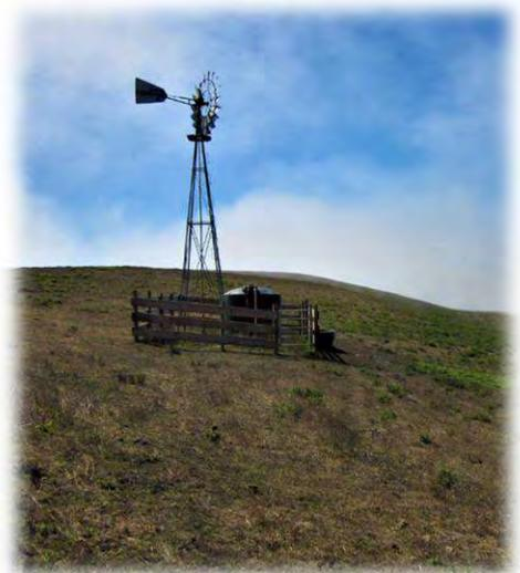
**Figure-5:** Windmill powered well located on the ridge along the southern property boundary. Well water is pumped into storage tanks and then flows via gravity to the Agricultural Lease area where water is provided to livestock in a number of water troughs.
